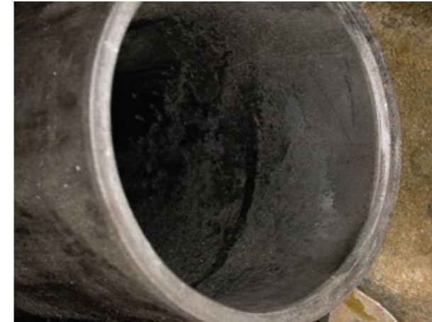
Figure 2: Valve guide with evidence of adhesion and abrasive wear [6].
